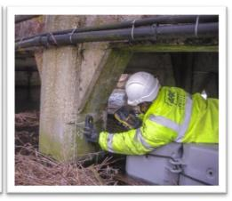
**The outcome:** The various surveys and testing carried out resulted in the generation of a report, detailing the findings of the defects survey, laboratory analysis and results, as well as recommendations for concrete repair and remedial works. Following completion of these surveying and testing works, Timsbury Bridge underwent a
